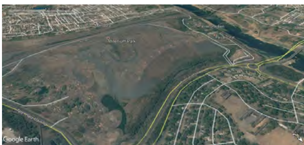
JMD before rehabilitation on April 2004
